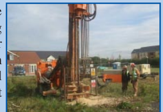
Pictured, piling works in progress at Bunkers Hill, Lincoln
