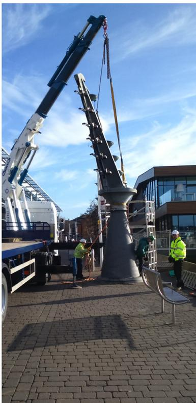
This well known Lincoln landmark features a 26' high rotating water clock that chimes on the hour. It hasn't worked for the past 10 years but that is all about to change as our Maintenance Department has taken it away to be refurbished and it will be back in its place during March and ready for the summer.
