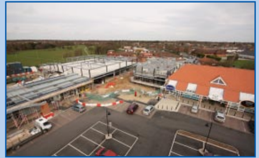
Pictured - an aerial shot of the development taking shape.
