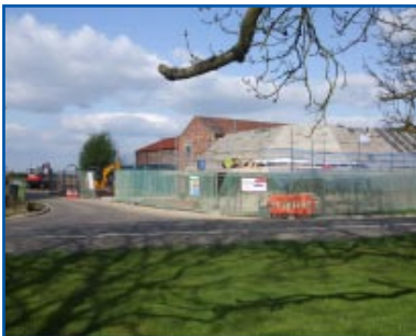
Pictured - the new office development taking shape.
