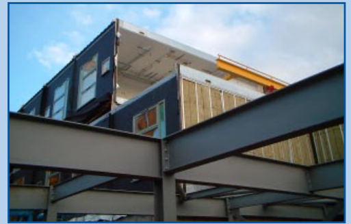
Works progress with some of the 56 modules being lifted into position
